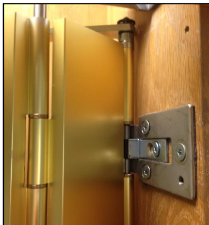
Figure 9 – Mounted hinge at the end of the half section.
